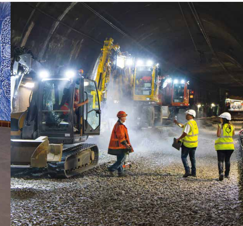
Paris Track upgrade on RER suburban line A
