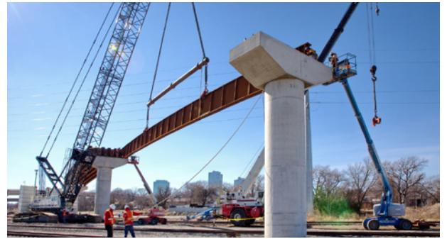
Peach Yard bridge construction north of Belknap Street
