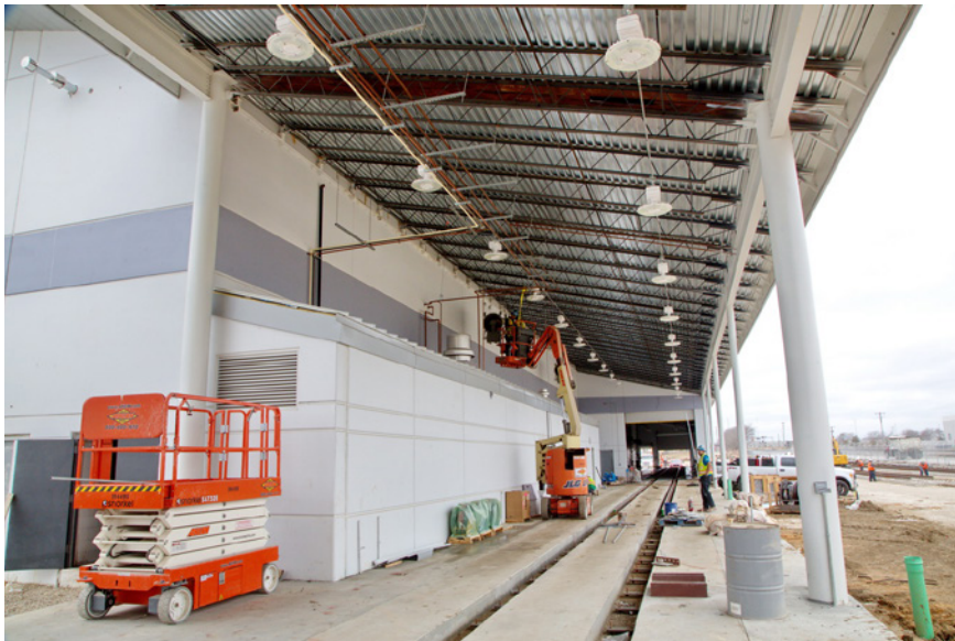
TEXRail EMF is nearing completion
