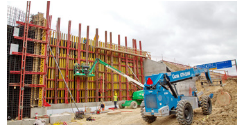
Construction at DFW Airport Terminal B Station
